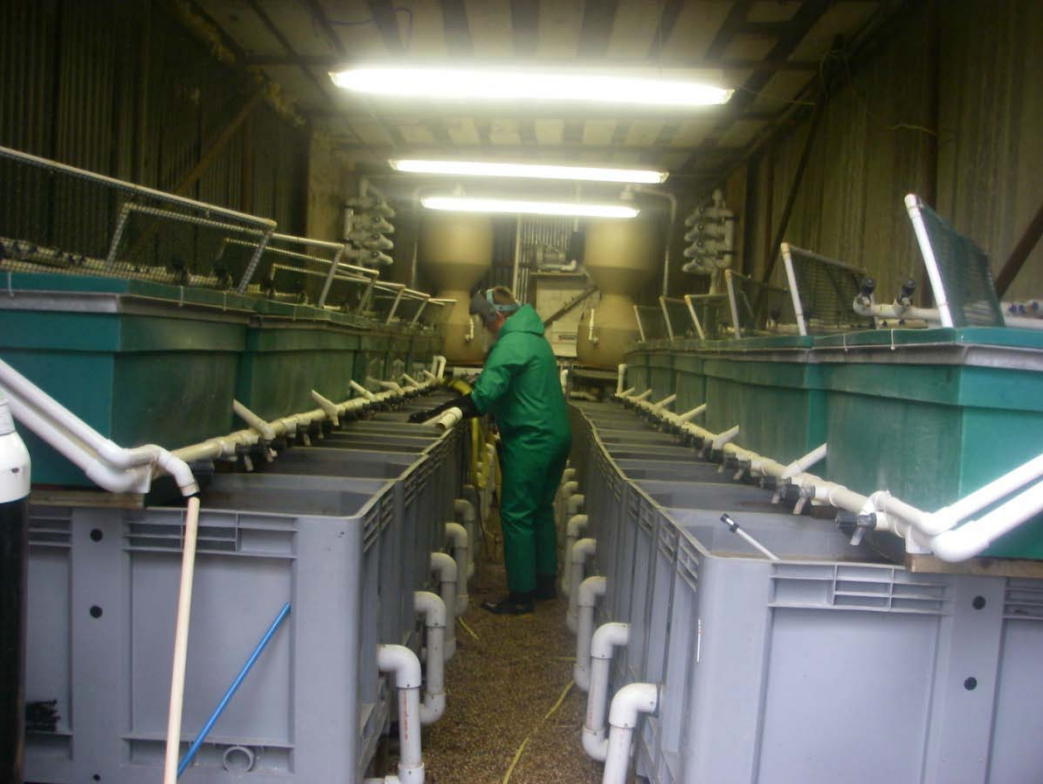
Photo 2 – Layout of recirculation systems
